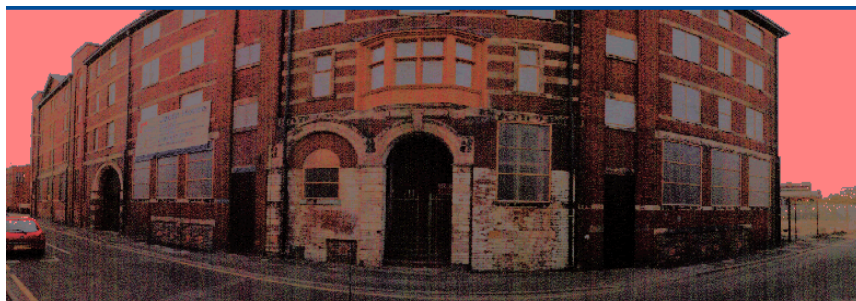
Figure 1: front point cloud image of the building based on the scanner field of view
