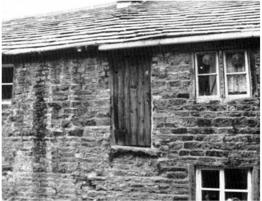
Figure 4b. Summerbottom rear taking-in door.
