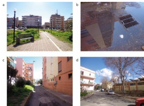
Fig. 1. Rione Marconi. (a) Open Space in the heart of the Area; (b) Damages to the sewage system; (c) Lack of maintenance; (d) School (Authors' photographs)
