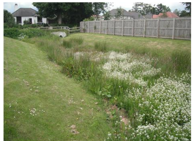
Fig. 1. SuDS swale with high macrophyte diversity adjacent to a green path, with cycling and pedestrian access at the back left of the image. Note the lack of barriers, other than where the path is immediately next to the SuDS. This site is used by local families for recreation and holds large breeding populations of common frogs ( Rana temporaria ) and palmate newts ( Lissotriton helveticus ). (Photo: D. O'Brien)
