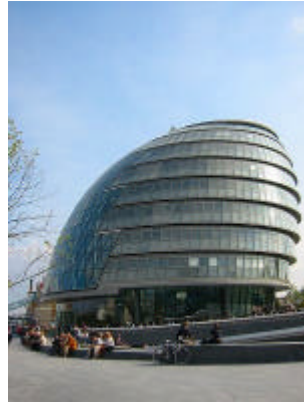
Fig. 3. Greater London Authority Building
