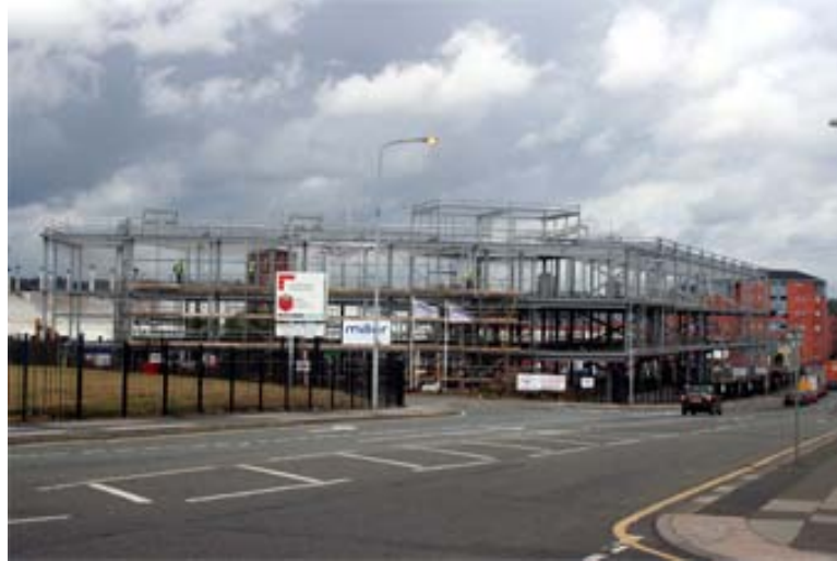
Figure 2 – New construction work on Frederick Road, Salford.
