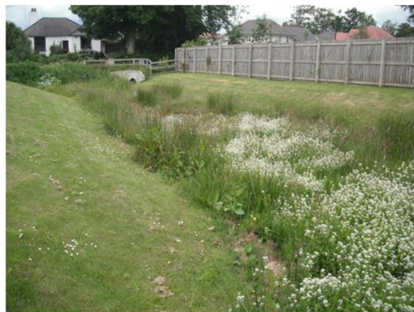
Fig. 1. SuDS swale with high macrophyte diversity adjacent to a green path, with cycling and pedestrian access at the back left of the image. Note the lack of barriers, other than where the path is immediately next to the SuDS. This site is used by local families for recreation and holds large breeding populations of common frogs ( Rana temporaria ) and palmate newts ( Lissotriton helveticus ). (Photo: D. O'Brien)
