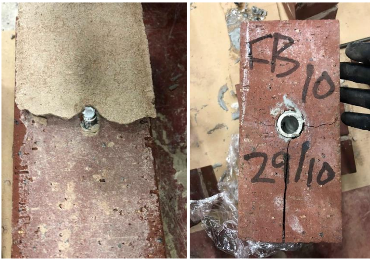
Fig. 5. Failure mechanisms identified in a) bar reinforced, and b) tube reinforced triplets [12].
